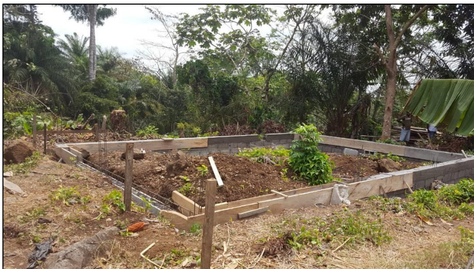
Foundations being laid for the quail farm
