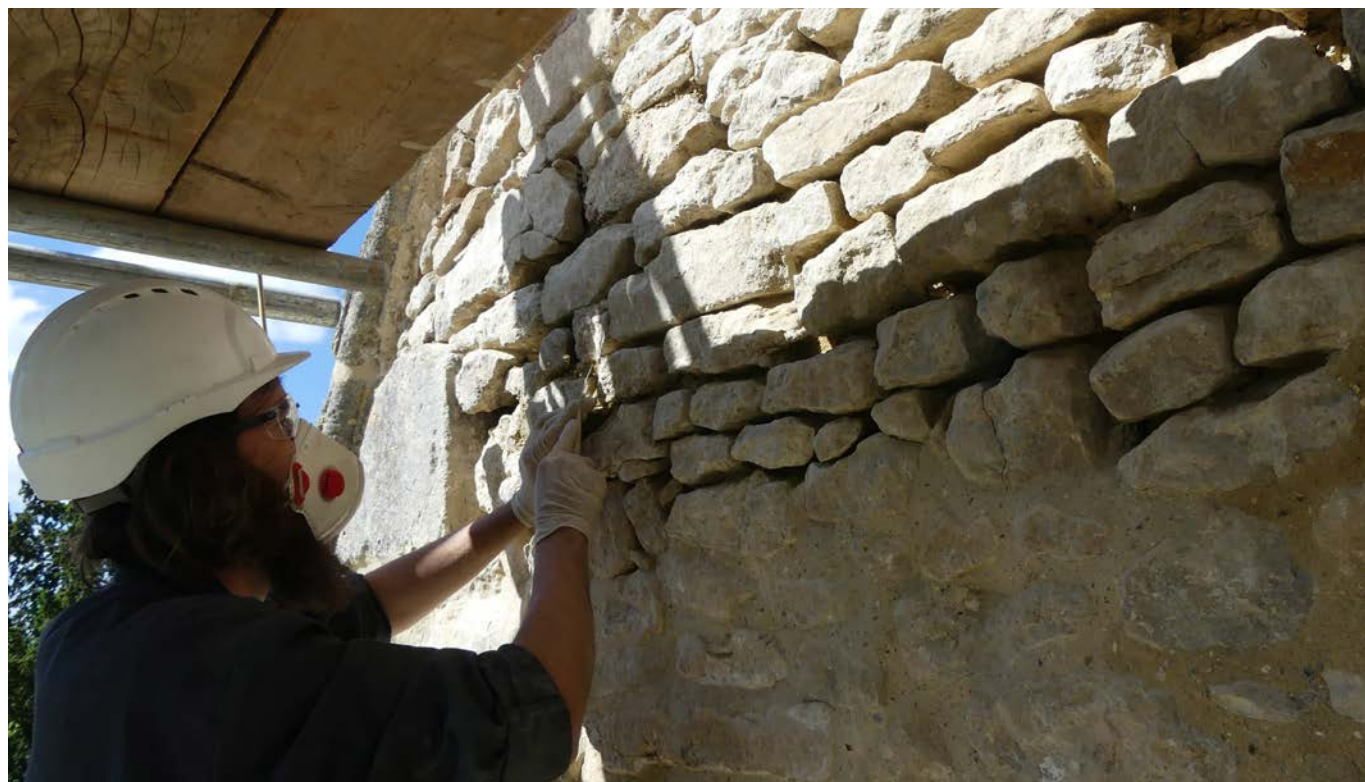
Stonework being repaired using lime mortar at St Mary's church, Long Crendon
