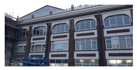
New concrete arches have been specially made and installed on the top row of windows and around the roof perimeter to match the design of the entrance.
