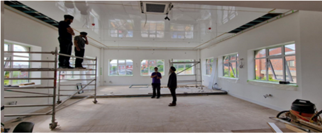
2nd floor Darbar in progress May 2022 (Wall panelling and AC system installed)
