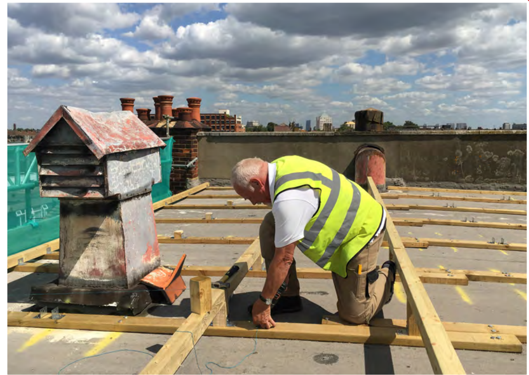
Temporary roof fitted to protect chapel by John Ryan
