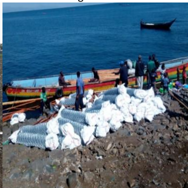
Fencing materials arrive
