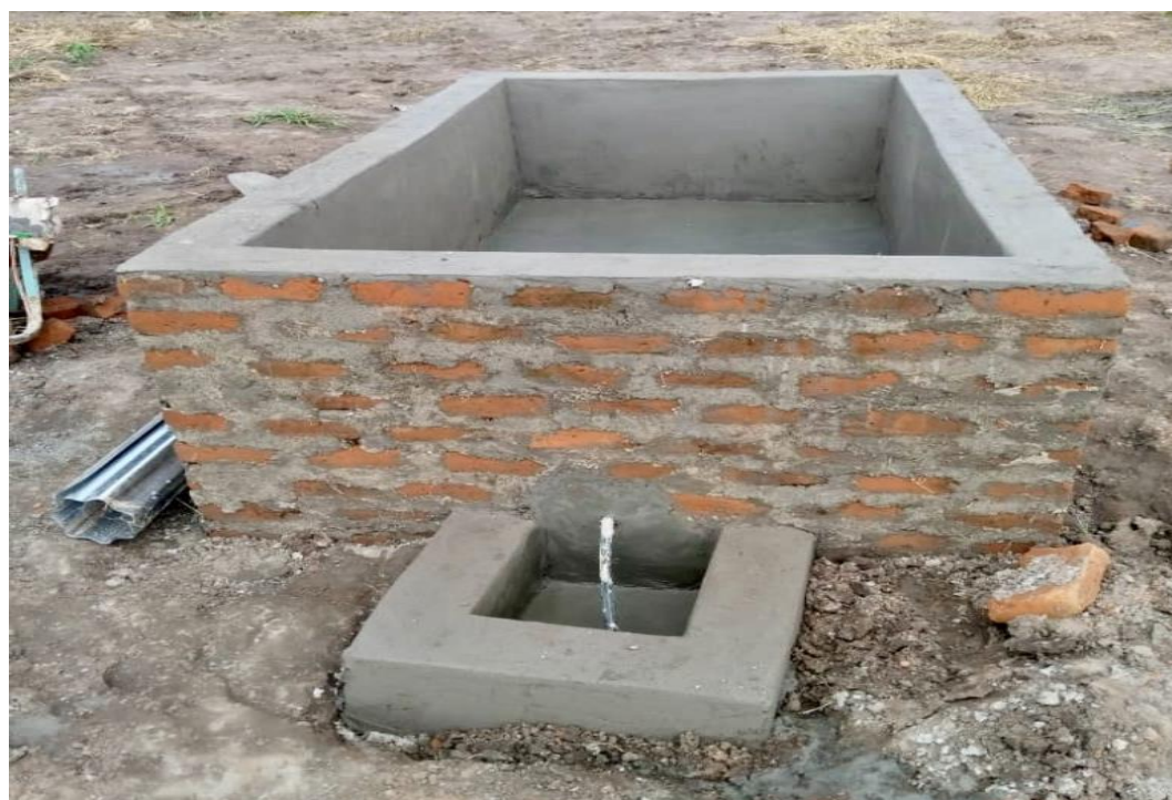
Building a vermiculture tank at Paorinher
