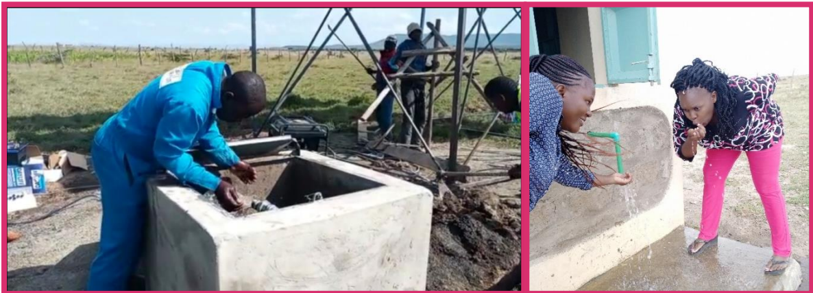
1. Installing the water solution
