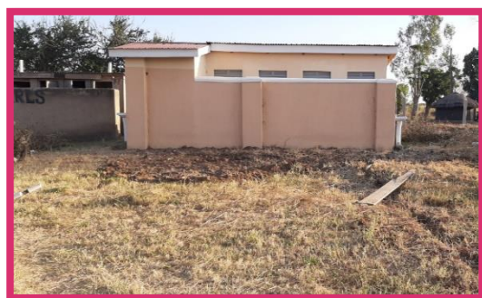
Washbasins have been installed as well as bio-toilets.
